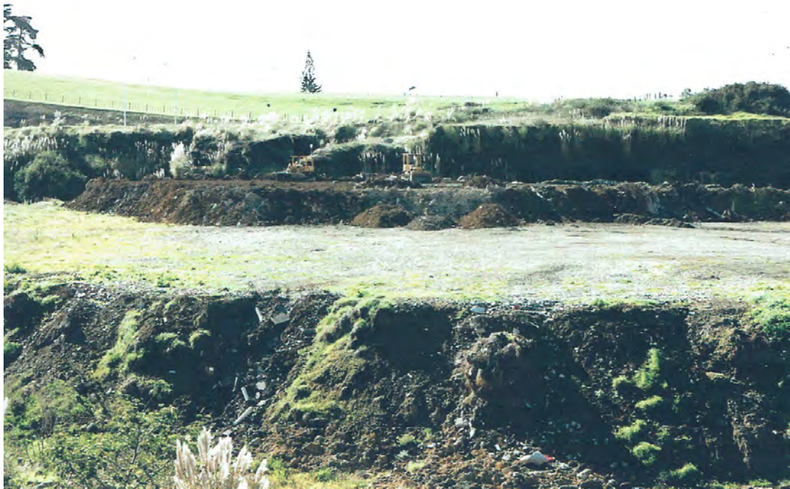
Figure 23: Filling of the quarry in progress in 2000. Photo: Self Family Trust.
