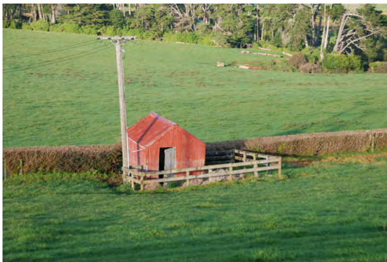
Figure 66: Pump shed on western slope of crater.
